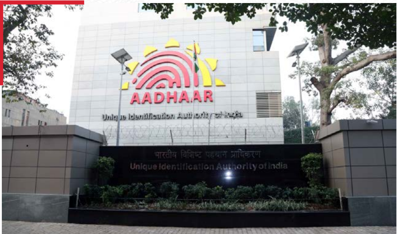
UIDAI Head Office Building, New Delhi
